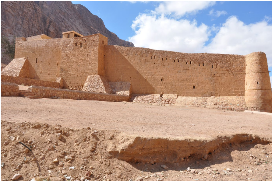
Fig. 1. View of the monastery’s eastern wall and “Round Tower” (Photo: Denis Nosnitsin)
